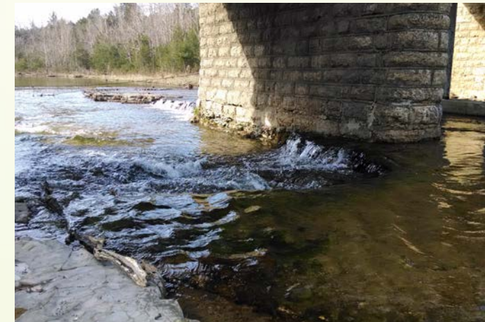
OFF HIGHWAY 201 | Stone County photo by: Paul Christenberry – Geotechnical Aide II
